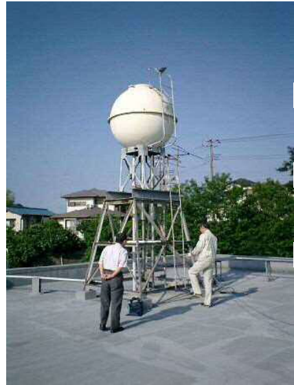
貯水槽の点検
