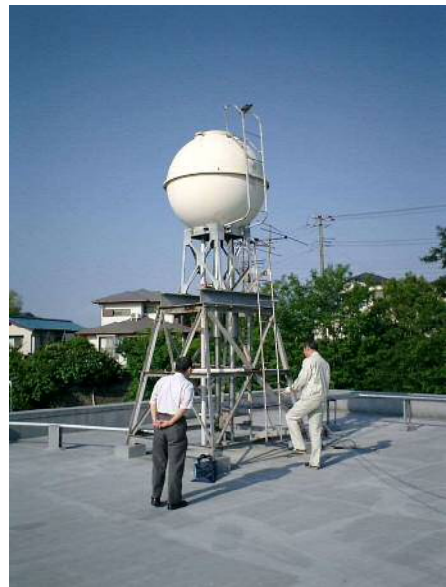
貯水槽の点検
